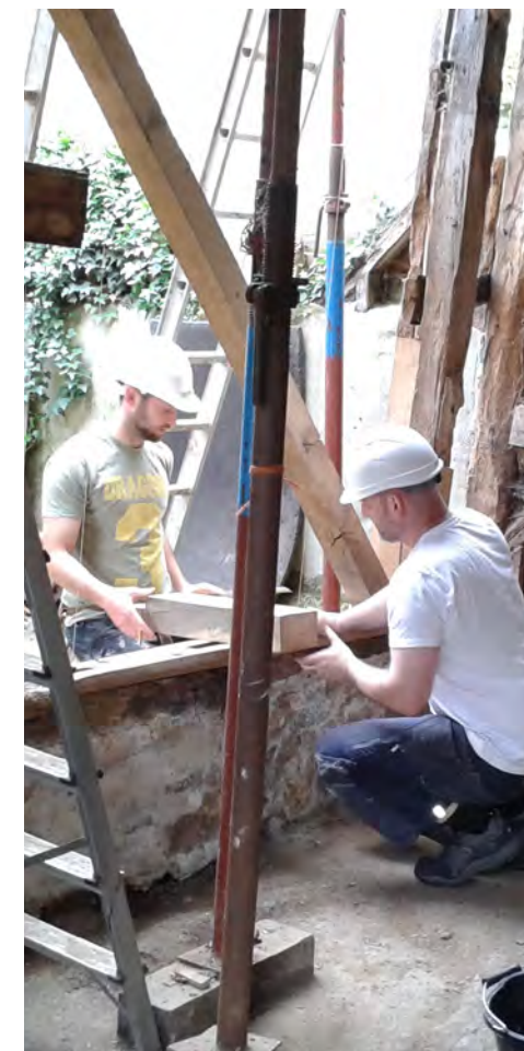
Educational training course on Timber Framing (ECC)
