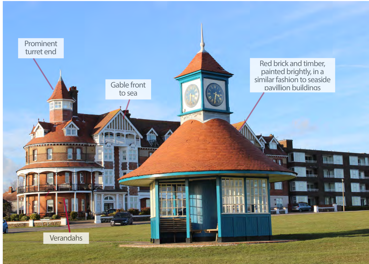
The Clock Tower shelter and former Grand Hotel, Frinton
